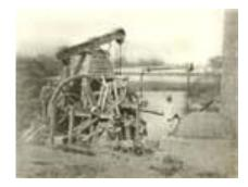
A Newcomen atmospheric engine was used for pumping water from mine
